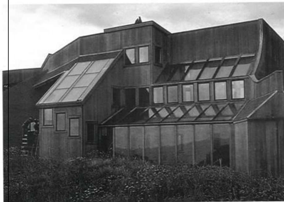
This solar home uses integrated solar water heaters to heat water and a photovoltaic array to generate electricity.
